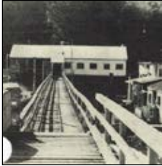
The Pier before renovations
